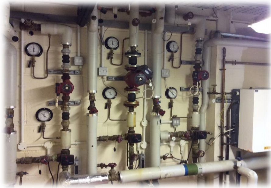
Image 4 - Variable Temperature Heating Circuits
