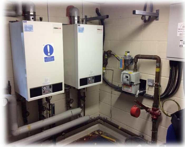
Image 3- Existing Boiler Plant and Gas Meter
